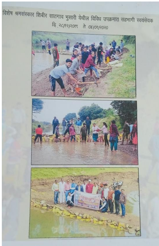
NSS volunteers constructed soil dam on river during 28/12/2019 to 04/01/2020
