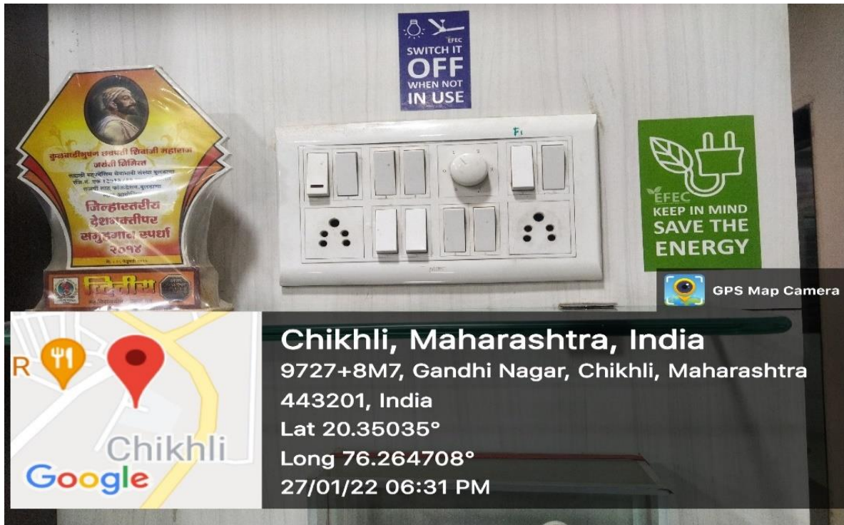
Save Energy Tips: Administrative office
