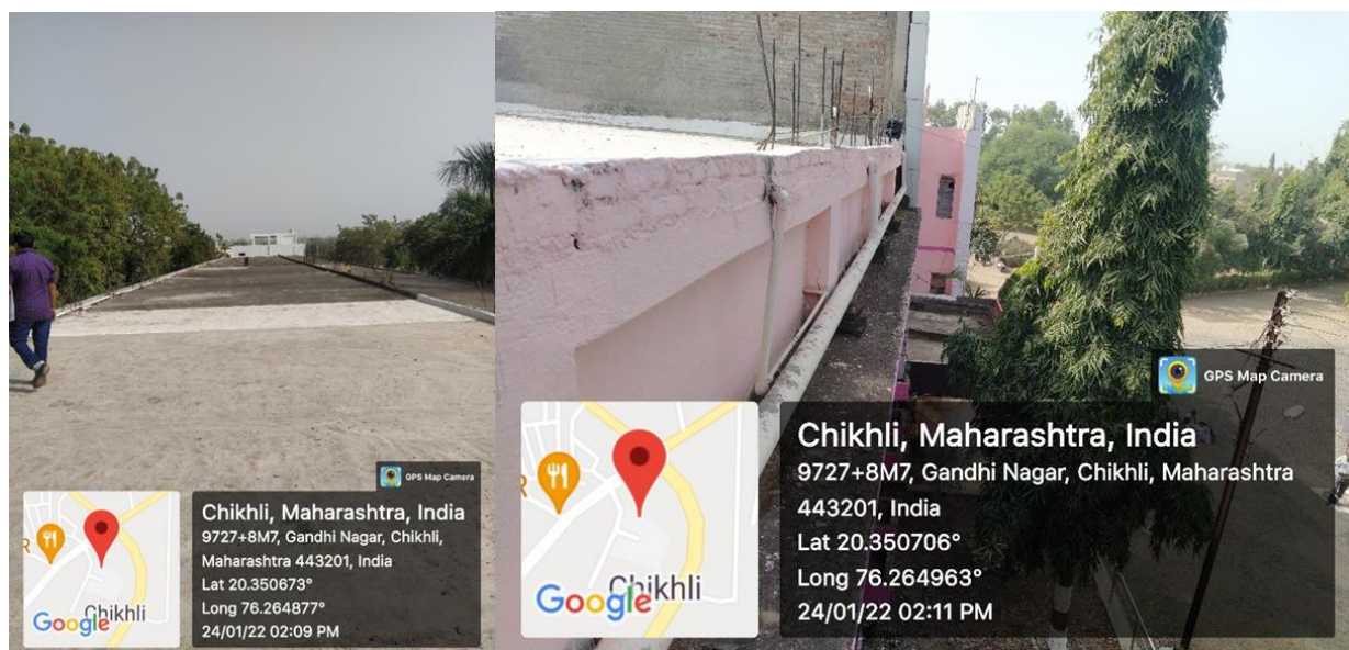
Water Conservation: Rooftop Rain Water Harvesting
