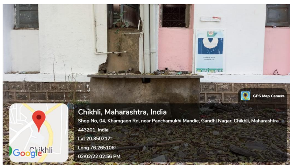
Liquid Waste Management: Facility for Chemistry Department
