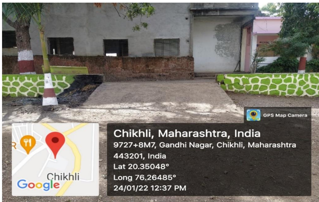
Divyangjan-Friendly, Barrier Free Environment: Ramp-1-For Seminar Hall/Classroom
