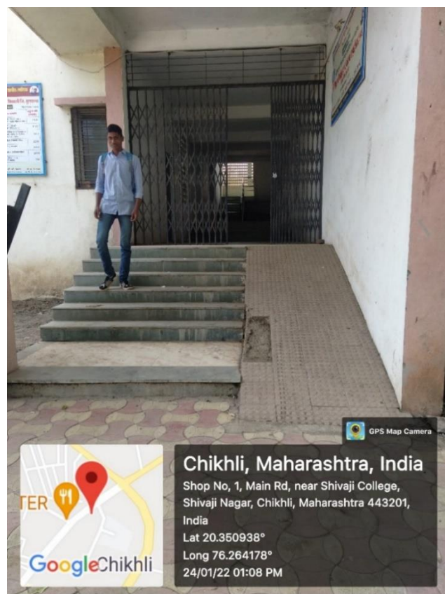
Divyangjan-Friendly, Barrier Free Environment: Ramp-4 for Girls Hostel & Open University Center
