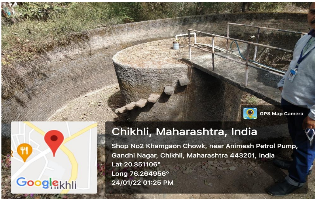
Composite Bore Well Recharge Project: Summer
