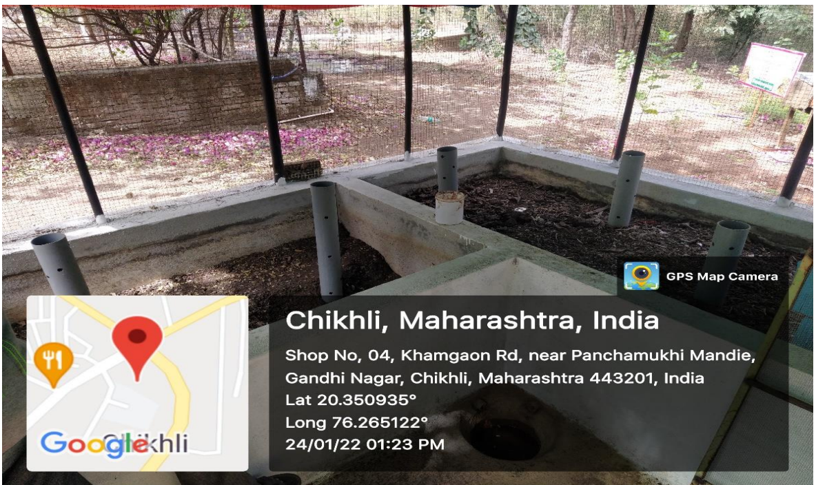
Solid Waste Management: Vermicompost Project for Organic Solid Waste
