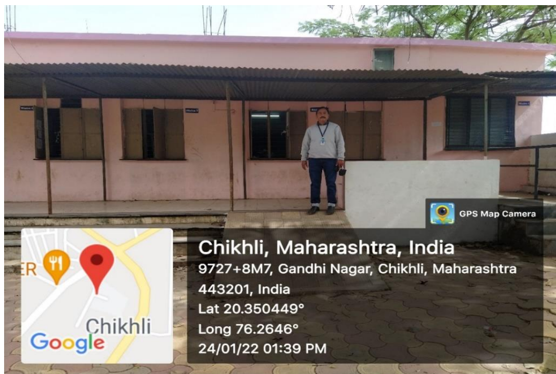
Divyangjan-Friendly, Barrier Free Environment: Ramp-2 for Administrative Wing
