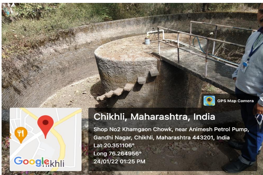
Composite bore well Recharge Project: Summer
