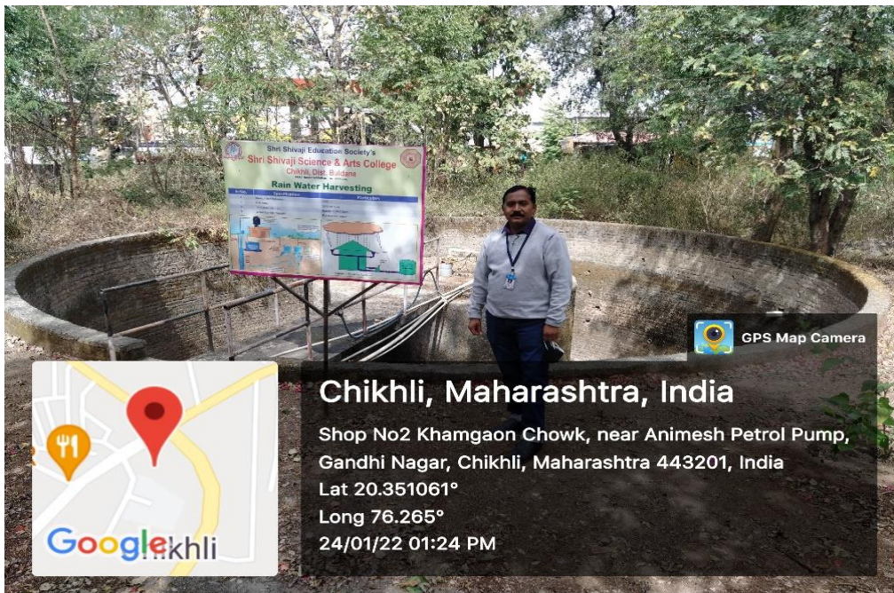
Composite bore well Recharge Project: Summer
