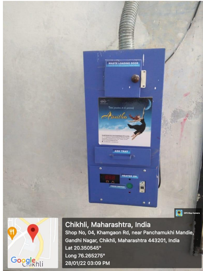
Girls Common Room: Sanitary Napkin Incinerating Machine
