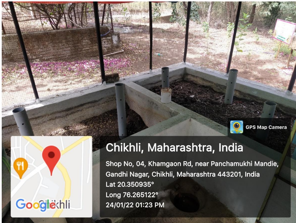
7.1.3/2 Solid Waste Management: Vermicompost Project for Organic Solid Waste
