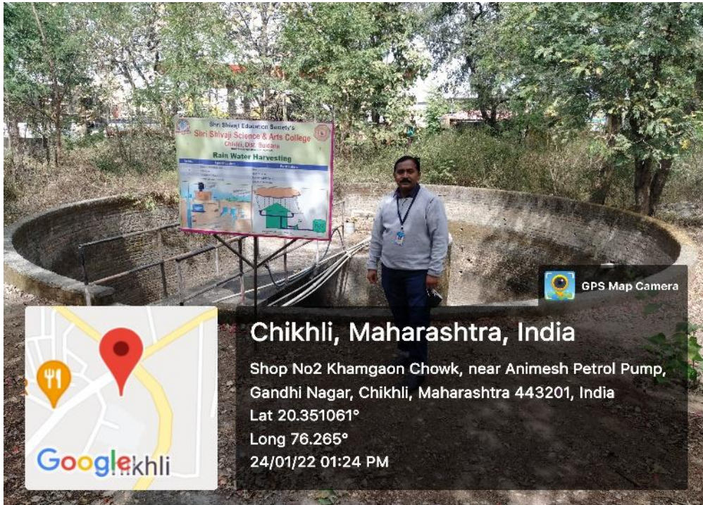
Artificial Borewell Recharge System (Before Monsoon)
