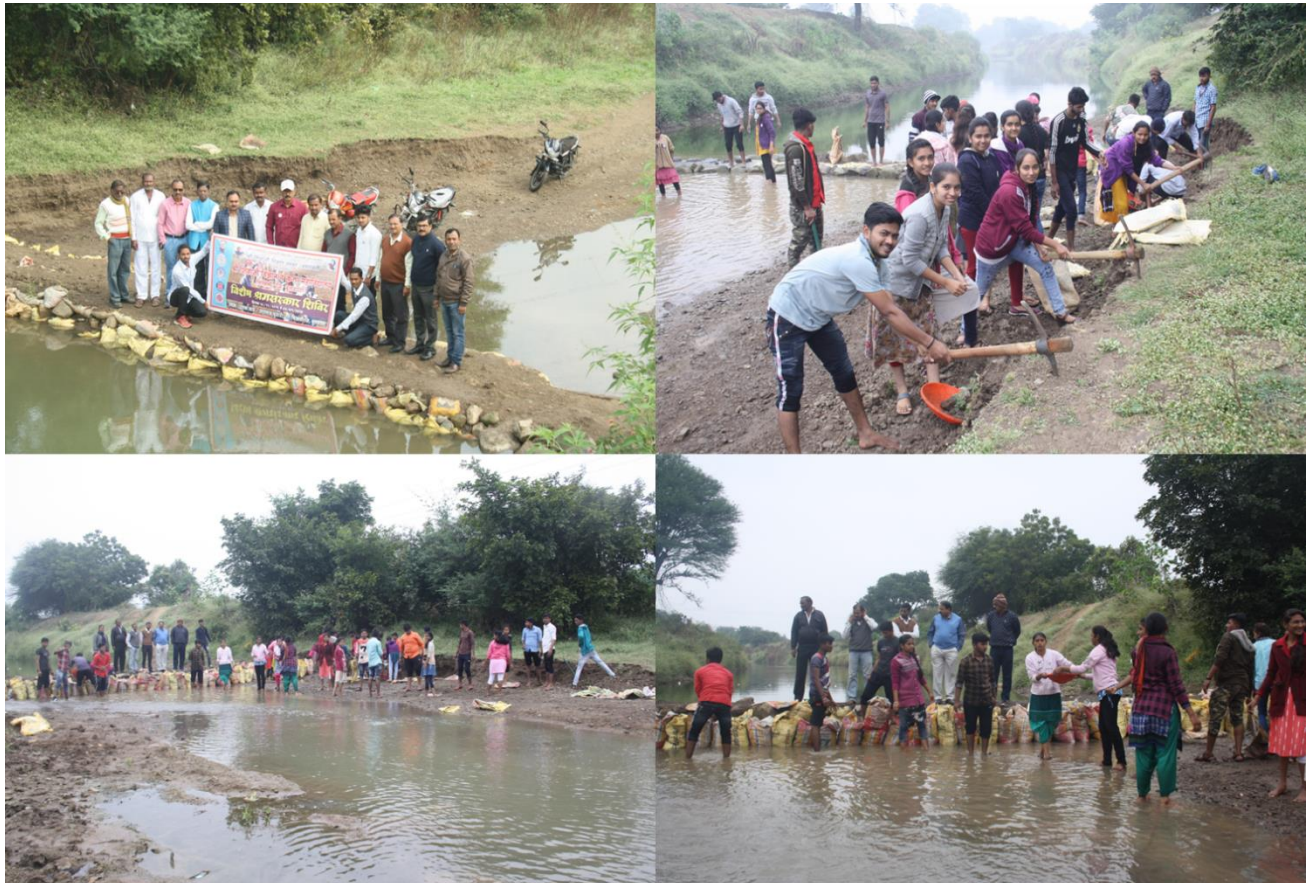
Bandhara Construction at Village Satgaon Bhusari Dist. Buldana: Students Contribution
