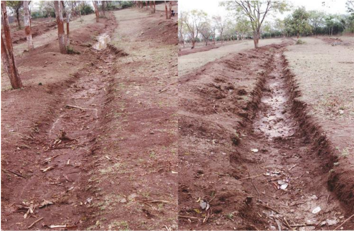
Recharge Trenches for Precipitation of Rain Water
