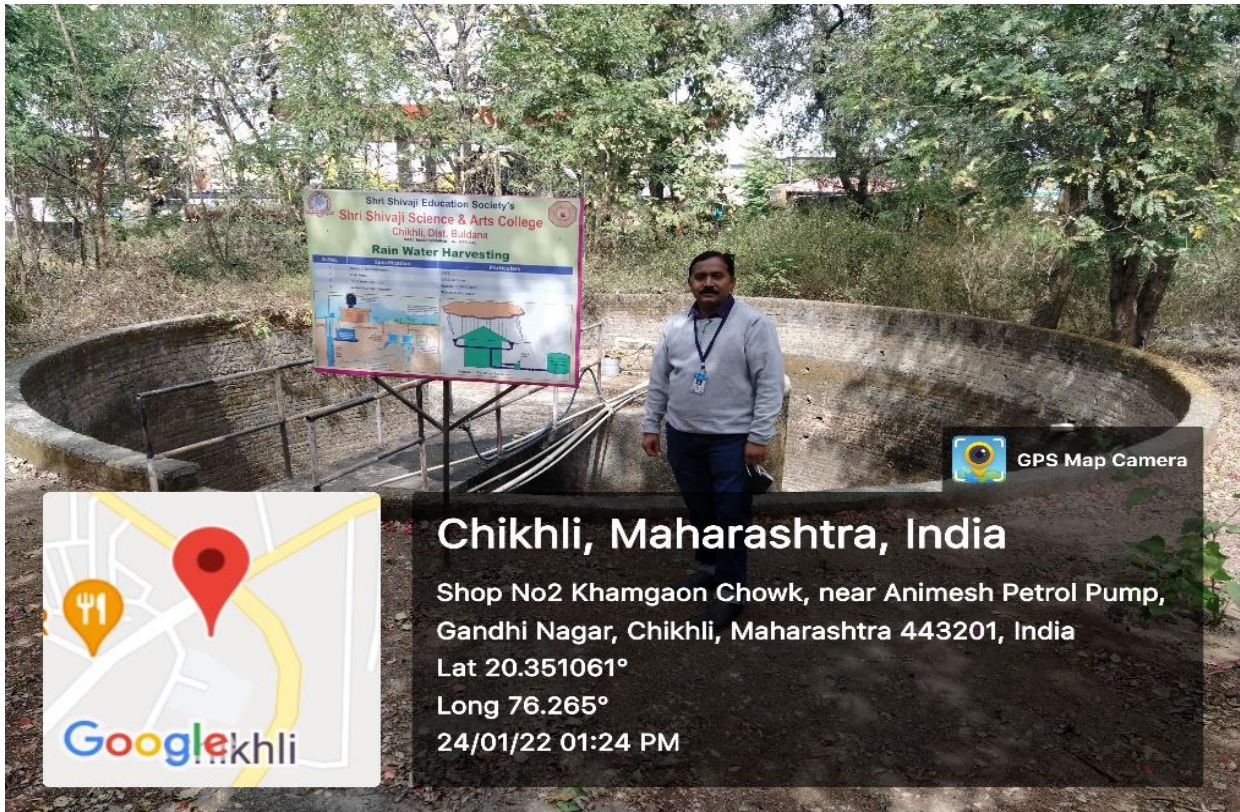
Composite bore well Recharge Project: Summer
