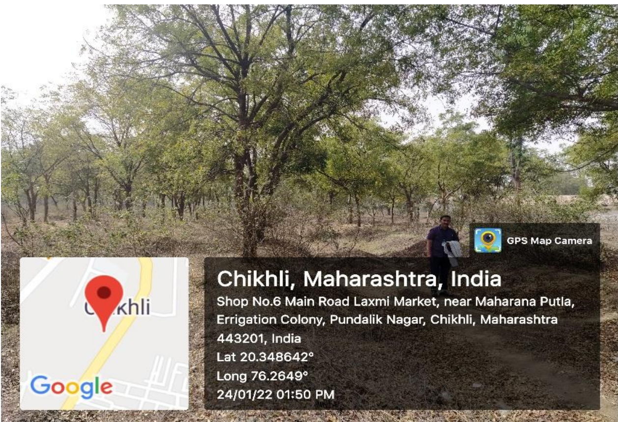
Recharge Trenches for Precipitation of Rain Water
