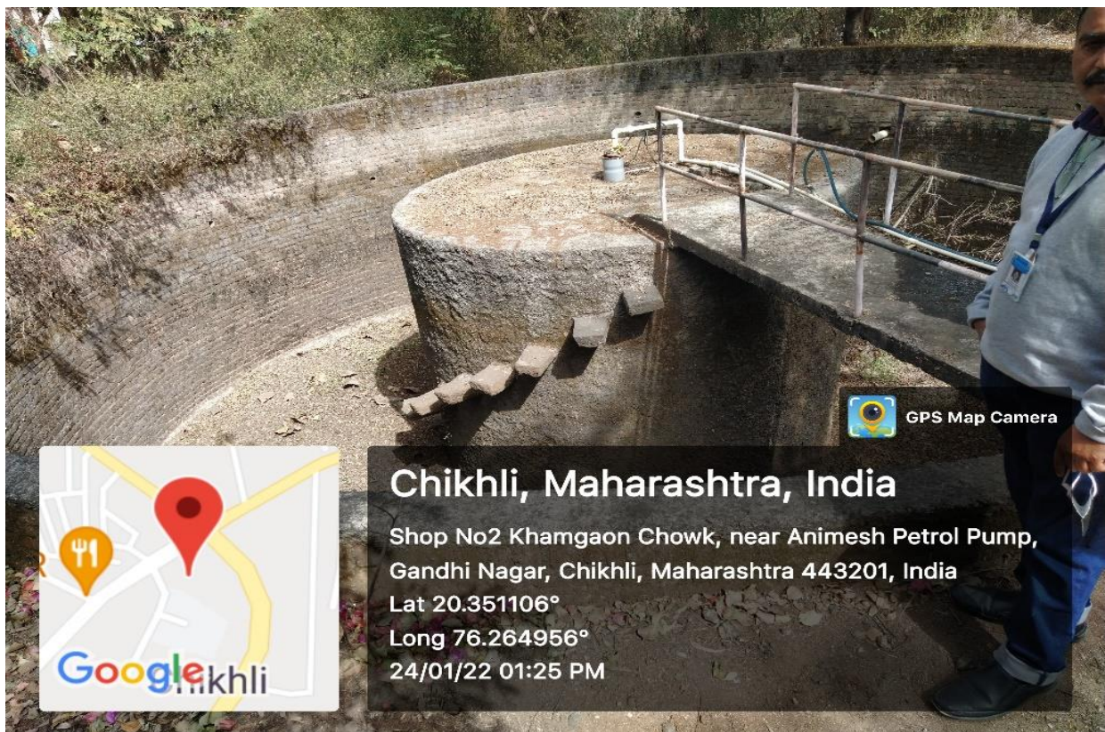
Composite bore well Recharge Project: Summer
