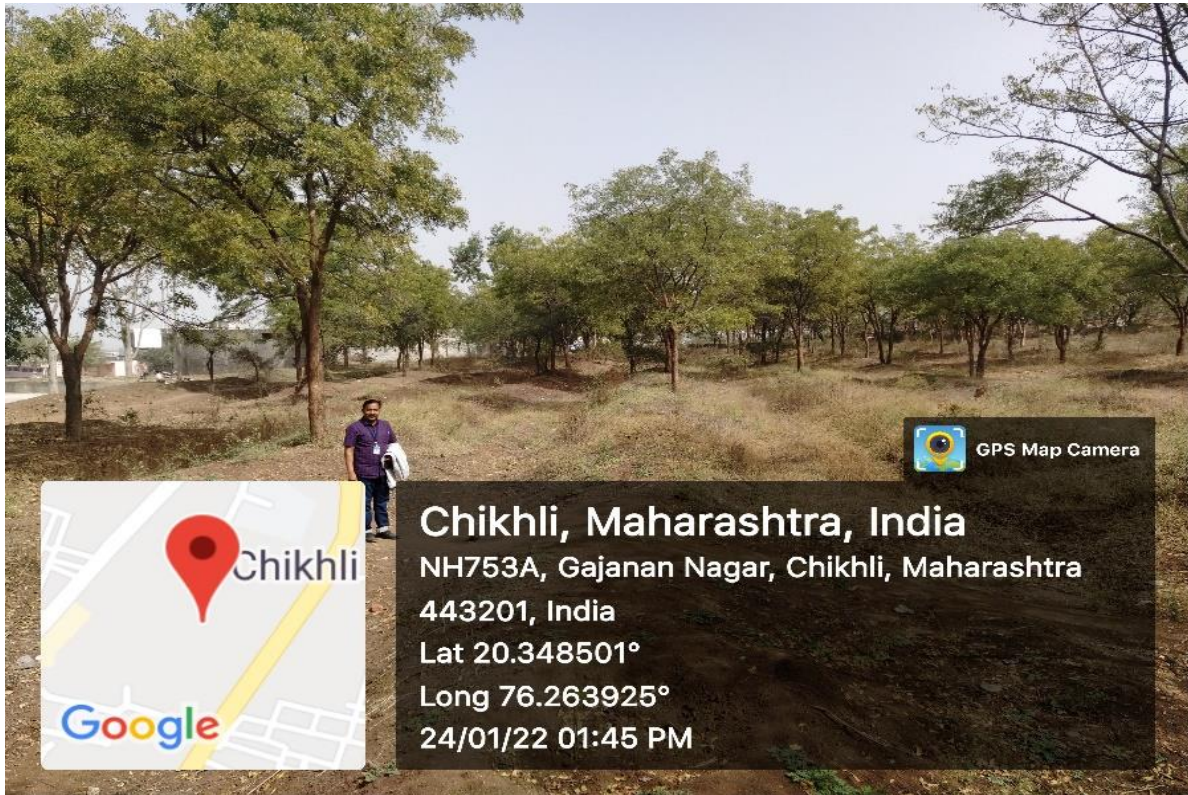
Recharge Trenches for Precipitation of Rain Water
