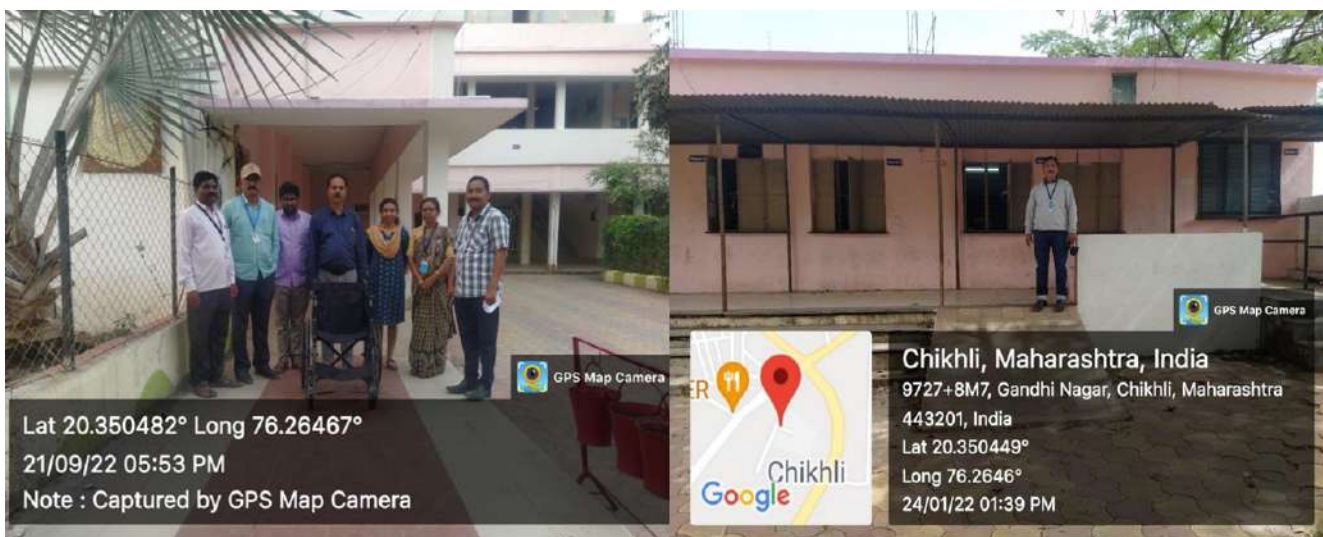
Divyangjan-Friendly, Barrier Free Environment: Wheel Chair & Ramp for Administrative Wing
