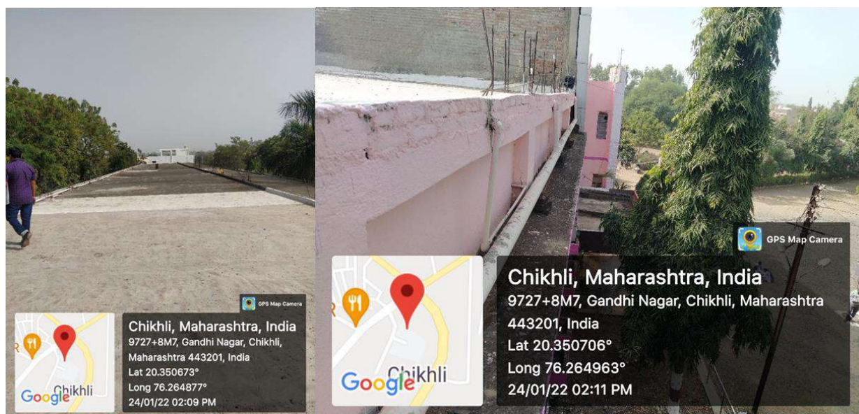
Water Conservation: Rooftop Rain Water Harvesting
